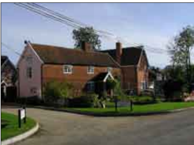
Willow Farm Cottage in 2005 - after the completion of the new housing development
